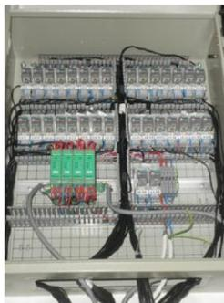
Figure 6. Relays connecting/disconnecting the controllable loads.
